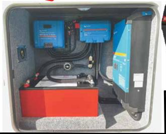
Lithionics 12V start and deep cycle 130 amp hour group 31 Lithium with built in Bluetooth. OUR Lithionics
